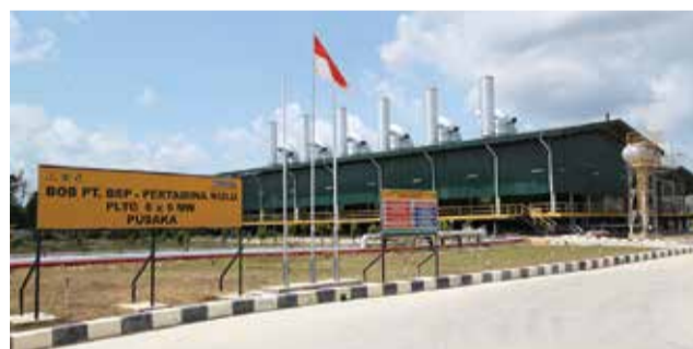
Fasilitas Power Plant BOB PHE-BSP, Riau.
